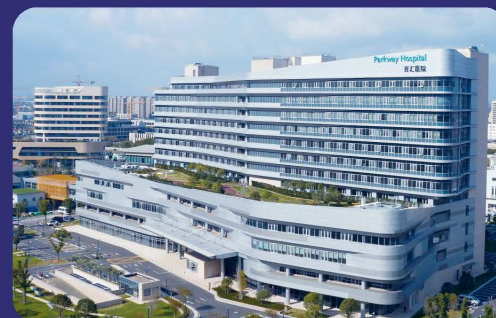
Parkway Shanghai Hospital
